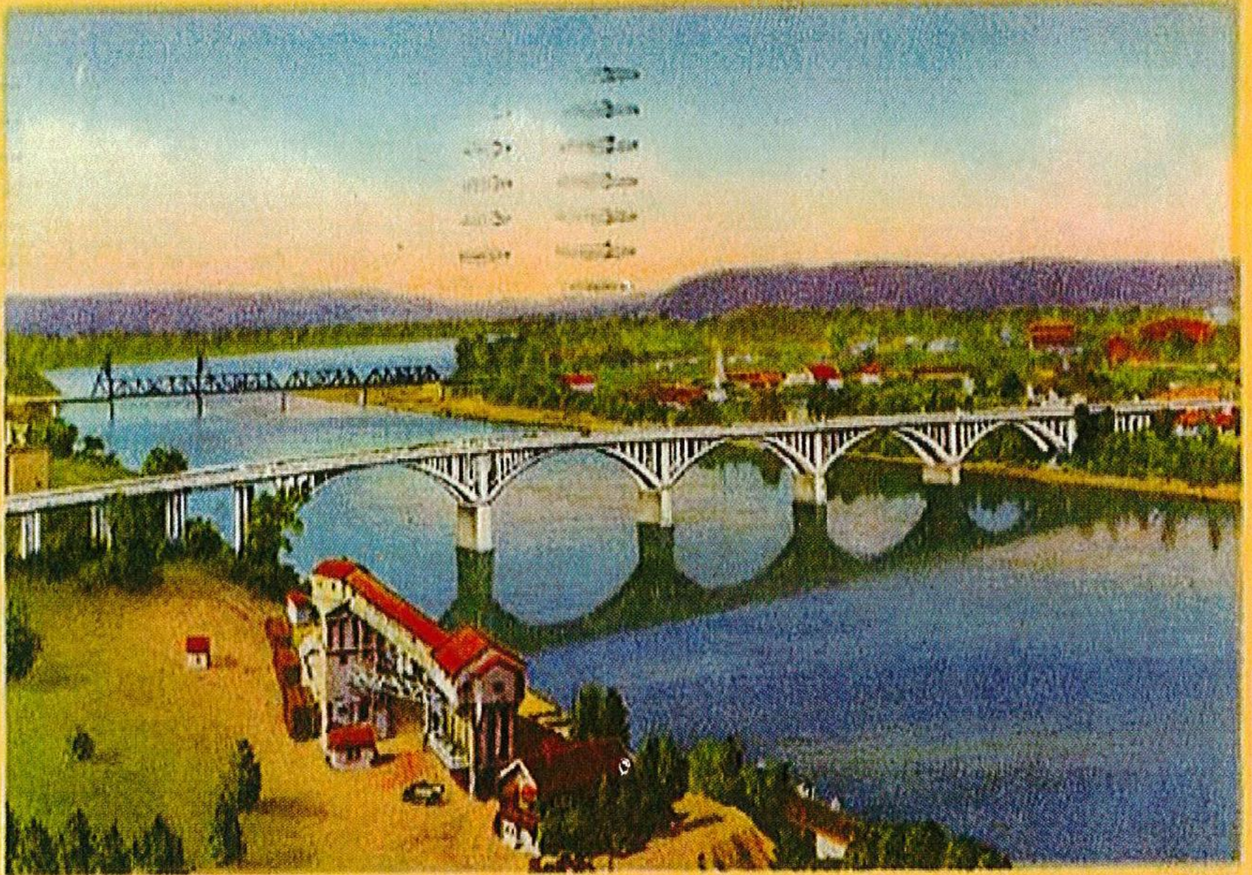
3—BROADWAY BRIDGE, LITTLE ROCK, ARK.
